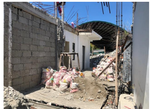
TWOP in San Jose—under construction!
